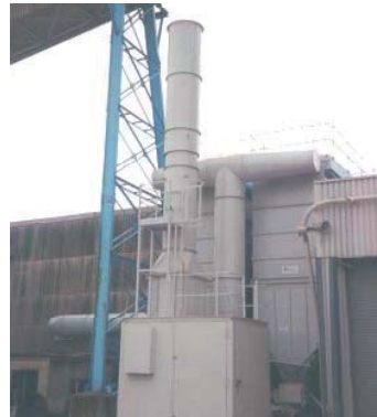
Cutting, trimming and finishing gypsum products
