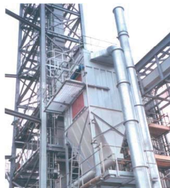
Dockside handling, conveying and storage, of grain
